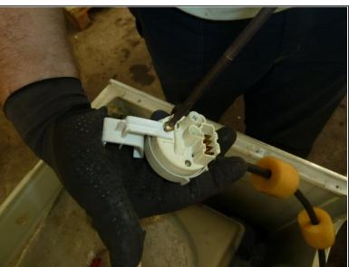
Unscrew and remove the pressure switch.
