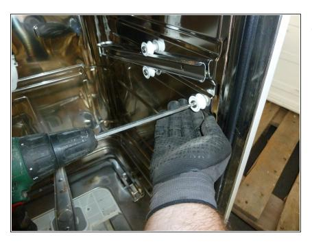
Unscrew the rails for the dish trays.
