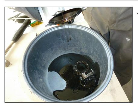
Remove the compressor oil by pouring into a safe container.
